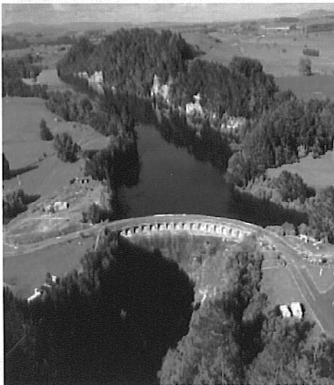
Figure 1. Arapuni Dam, New Zealand, looking West
